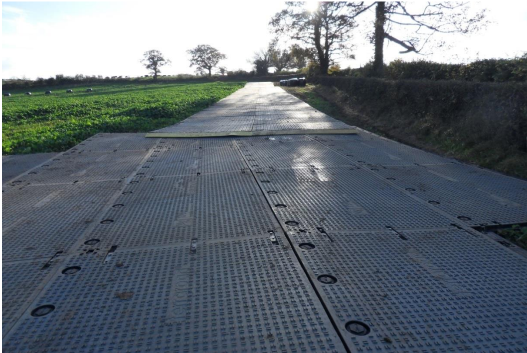
Figure 7.1 – Temporary Trackway.
